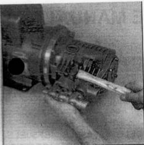
Removal of Discharge Manifold
